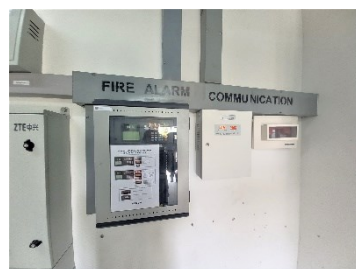
Fire Alarm Control Panel
